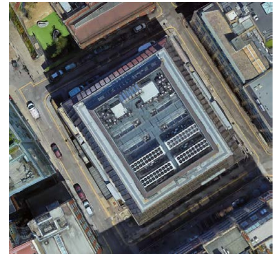
Figure: Volta Data Centre
